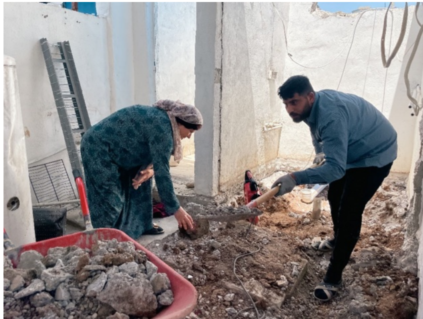
Shelter upgrades in Domiz 2
