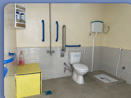
Improvements of latrine and shower (before and after) which includes constructing handrails, shower and shower seats, as well as accessible latrine, increase the safety of persons with disabilities and elderly.
